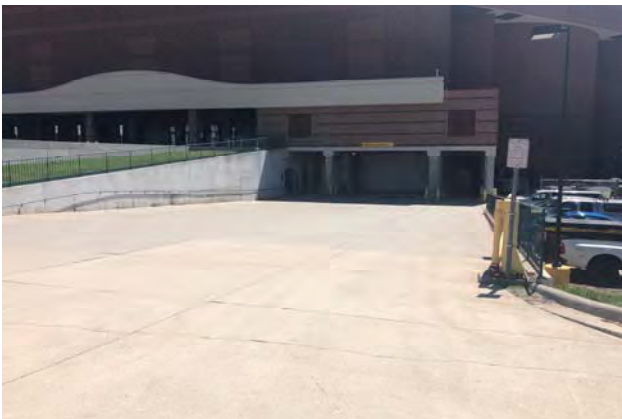
Figure 5. Loading Dock Ramp located on North end of building.
